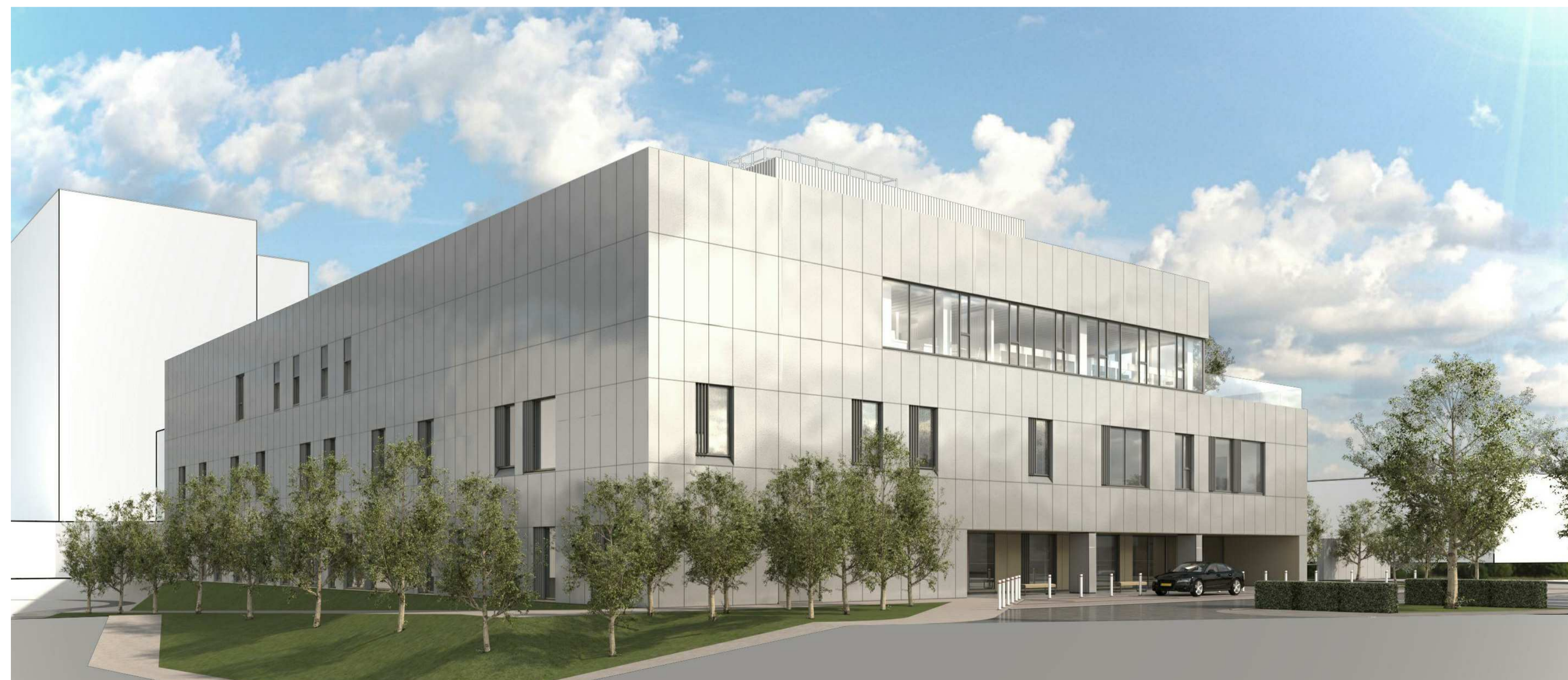
Entrance From South
