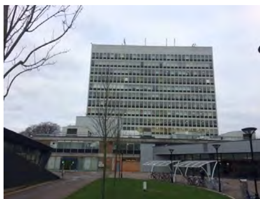
Figure 2 – VHK Tower Block
