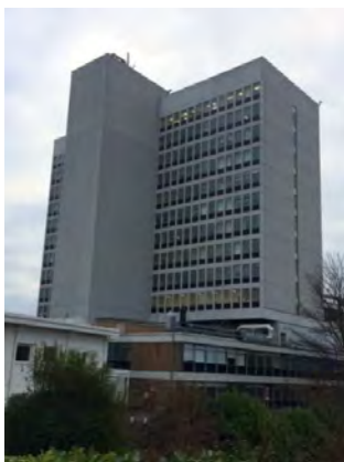
Figure 1 – VHK Tower Block
