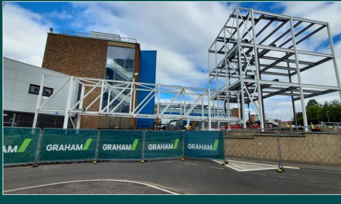
Erection of Steel Frame
