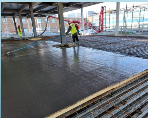
Concrete Floors being poured
