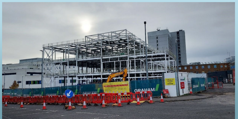
Steel Frame completion
